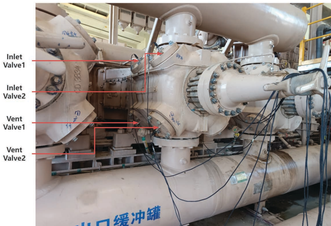
Figure 1. Location map of vibration signal acquisition points for the air valve.
